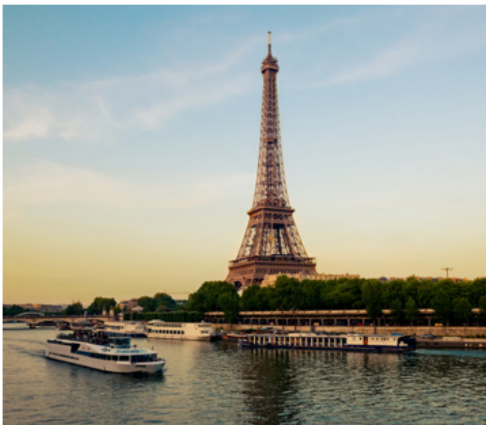
EIFFEL TOWER ACROSS THE SEINE RIVER
